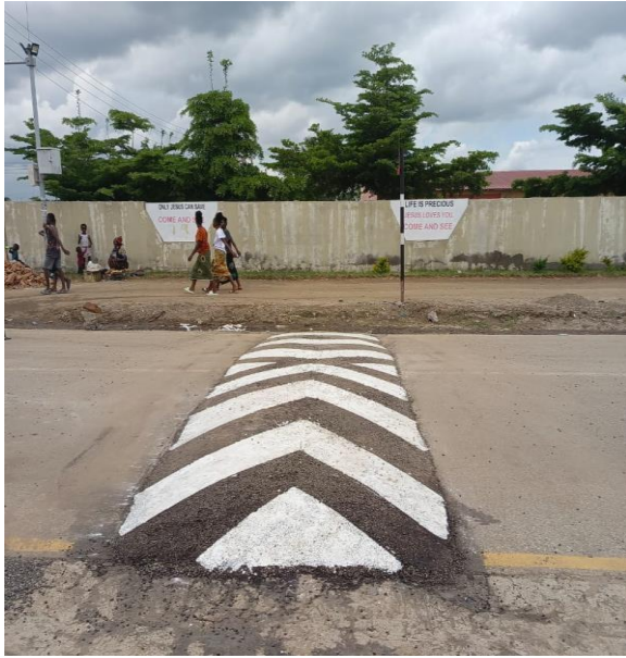
Figure 5. A new speed hump outside Kizito Primary School and a sign to warn vehicle drivers. Photo: Somela Sinkala.
